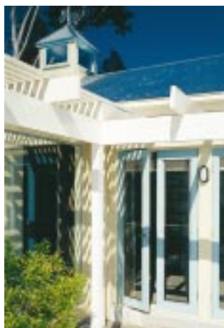
Sashless windows installed into doors.
